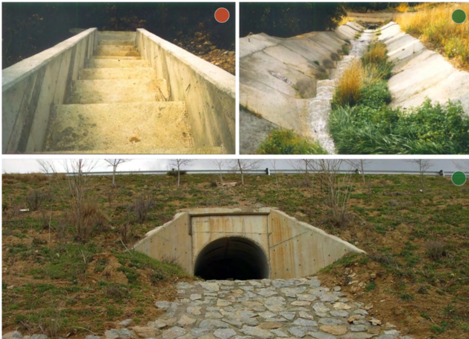
Figure 7.4.43 – A stepped drainage exit with vertical walls can trap animals and must be avoided. Opening the lateral walls of the channel or substituting the steps for a ramp with a rough surface will allow fauna to reach the embankments and access areas adjacent to the infrastructure. (Photos by: Minuartia).
