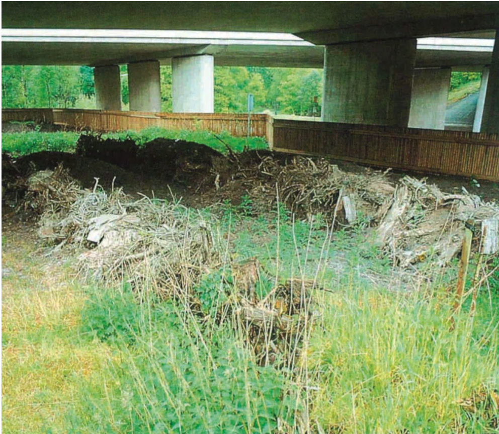
Figure 7.4.28 – Tree stumps were used as shelter for animals under the Zandheuveld viaduct on the A27 in the Netherlands. The wooden screen separates a road under the viaduct from the wildlife passage to reduce traffic noise and light disturbance (Photo by: H. Bekker).
