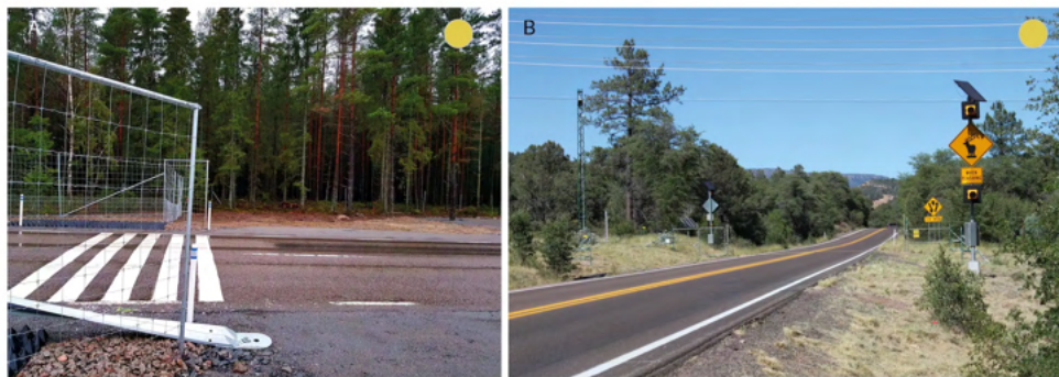
Figure 7.4.59 – Complementary warning measures to drivers improve the efficiency of at grade passages. A: White lines help animals to be seen on the road (Photo by: M. Elfström – EnviroPlanning AB); B: ADS warning signs installed with an at grade passage are activated when an animal is detected on or near the causeway (Photo by: C. Rosell).
