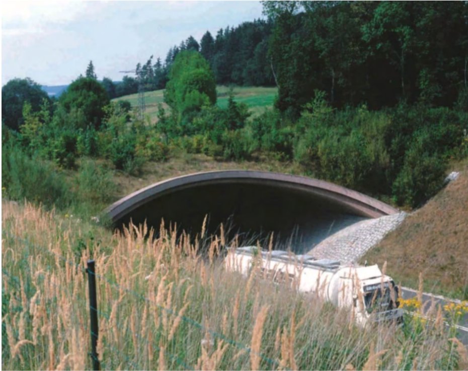
Figure 7.4.6 – A landscape overpass (50 m wide) densely covered with bushes and small trees since it aims to connect the adjacent forests on the B31, Schwarzgraben, Germany (Photo by: V. Keller).
