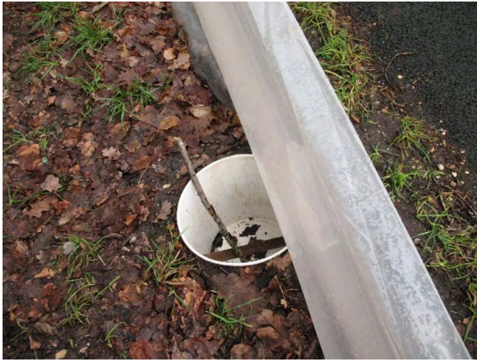
Figure 7.4.56 – Temporary amphibian fencing and buckets installed at the intersection of a migration corridor where animals can be collected and transported to the other side of the transport infrastructure (Photo by: C. Rosell).
