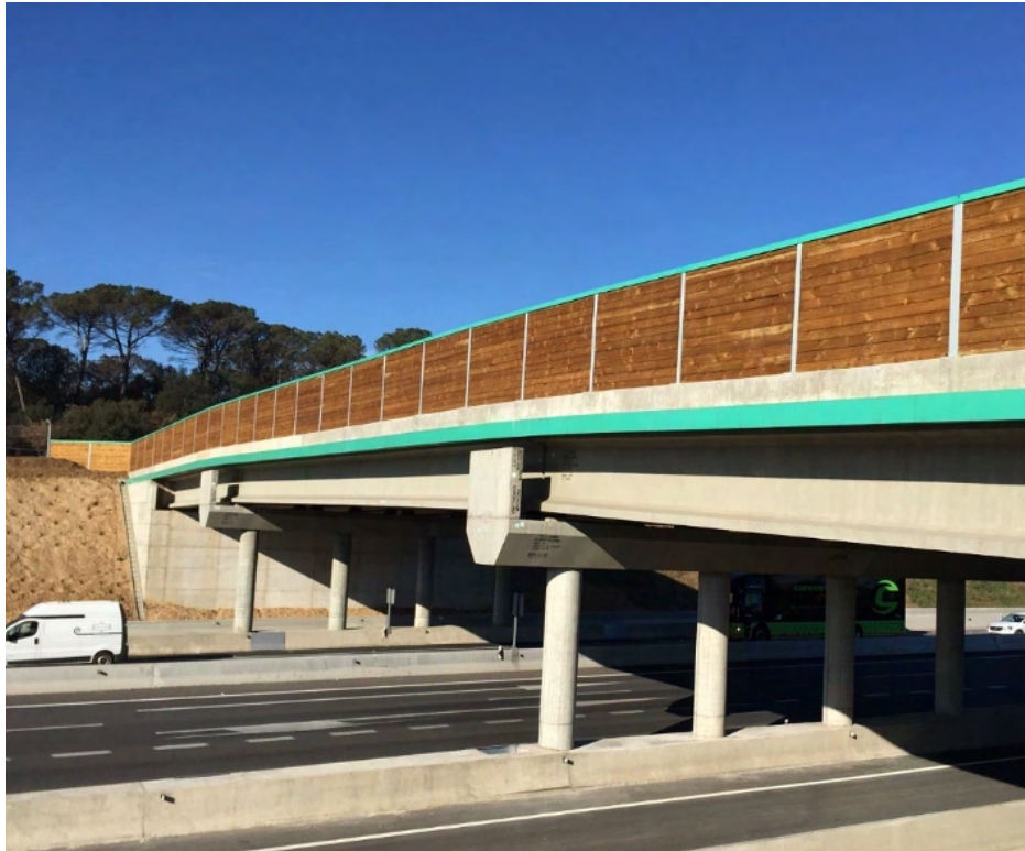
Figure 7.4.8 – Screening reduces disturbance from light and noise on the wildlife overpass. Materials should be durable and well-integrated. Systems to reduce vandalism could be installed, such as the upper metal barrier at the top of this screen on the A2 in Catalonia, Spain. (Photo by: Minuartia).
