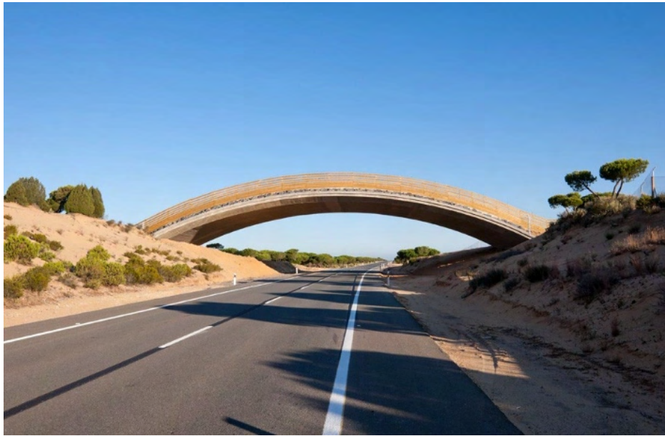
Figure 7.4.16 – Wildlife overpass designed as an arched platform without pillars, reducing the amount of materials used while ensuring an appropriate height to allow circulation of trucks on the A483 in Andalusia, Spain (Photo by: Agency of Public Works, Andalusian Government).
