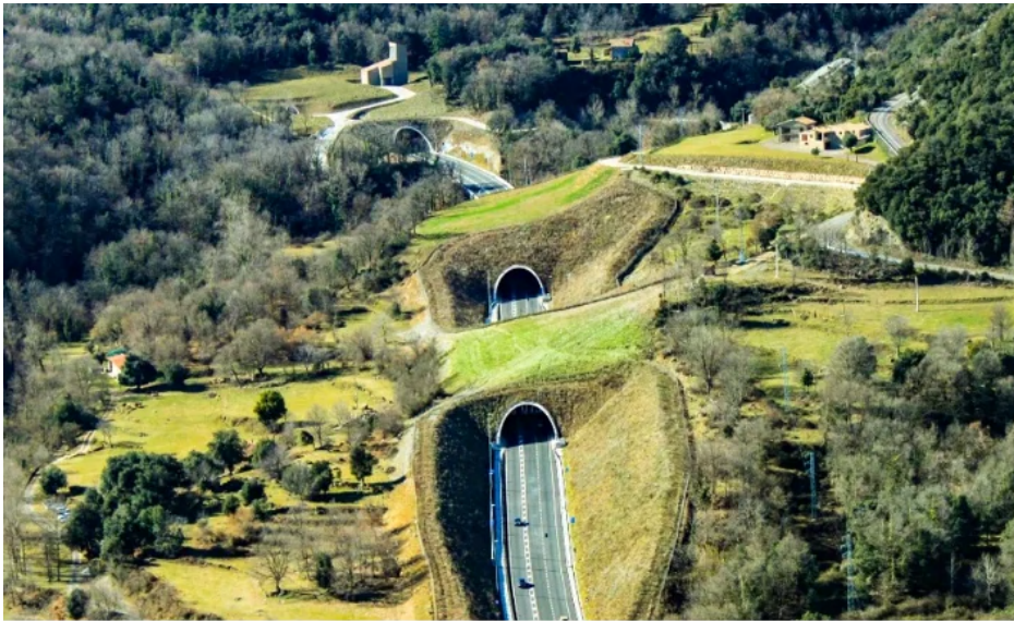
Figure 7.4.15 – Wildlife overpasses constructed by cut-and-cover tunnels providing links for pasture habitats. (Photo by: C. Rosell).
