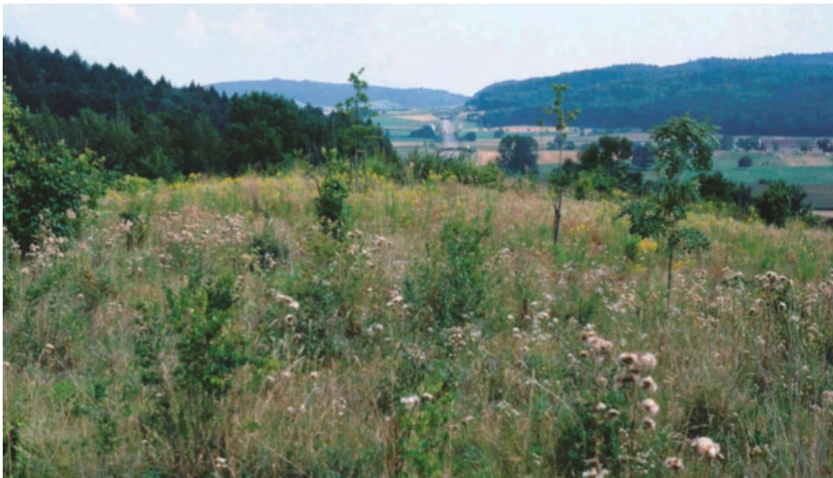
Figure 7.4.7 – Landscape overpass (80 m wide) where only bushes were planted while spontaneous growth of herbs and grasses was allowed, which may be later managed by mowing or grazing, on the B31, Weiherholz, Germany (Photo by: V. Keller).
