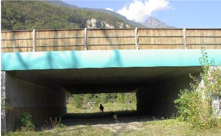
Figure 7.4.32 – Wildlife underpass in France with visual screens to reduce light disturbance from traffic. (Photo: C. Rosell).
