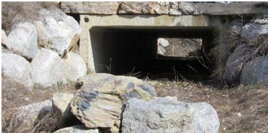
Figure 7.4.39 – Small fauna underpass constructed under an existing road to provide a safe crossing point for otters. Stones piles provide extra shelters. (Photo by: Minuartia).
