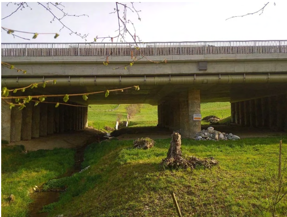
Figure 7.4.37 – Multiuse underpass that combines the crossing of a stream (drainage function) with wildlife use. Piles of stones and branches provide refuges for small fauna (Photo by: A. Righetti).
