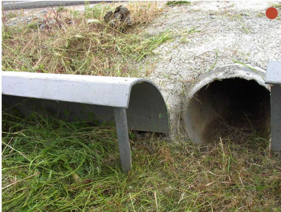
Figure 7.4.53 – Fencing must facilitate vegetation maintenance tasks and should be completely anchored to the entrance of the road. Red circle : vegetation, Yellow circle : access to road, Green circle : amphibians may access the road (Photo by: Minuartia).
