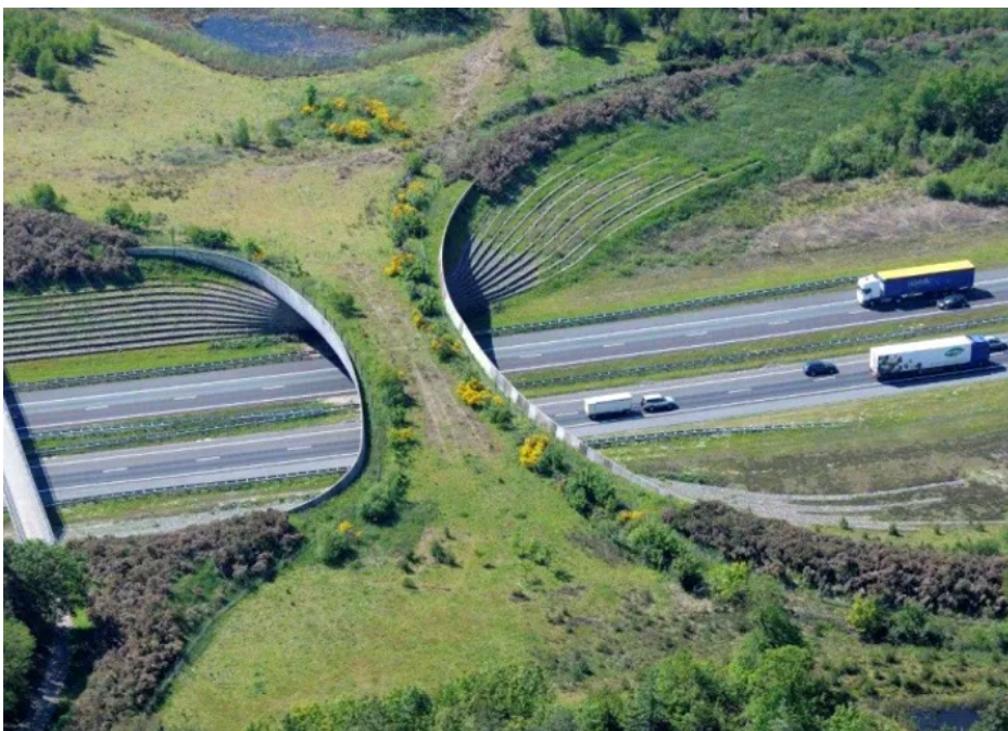
Figure 7.4.10 – An hour-glass shape maximizes width at the passage entrance. Different landscape elements (a pond, open grasslands, bushes) maximize the number of species attracted to this ecoduct on the N69 in Borkel, The Netherlands (Photo by: Geo Dienst – Rijkswaterstaat).
