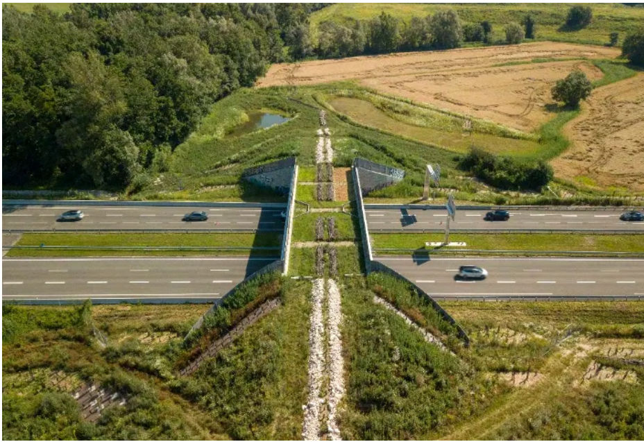
Figure 7.4.9 – Wildlife overpass in France, where the passage is accessed by ramps (Photo by: R. Couteau – AREA).
