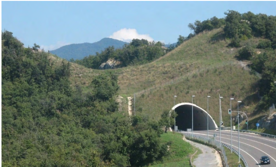
Figure 7.4.11 – Shaping the surface of a landscape overpass with a topography similar to its surroundings allows a variety of slopes and orientations increasing diversity of habitat conditions provided to invertebrates and small vertebrates as shown by this overpass on the C37 in Catalonia, Spain (Photo by: Minuartia).
