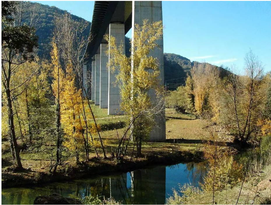
Figure 7.4.27 – A river crossing which preserves the natural riverbed and also the riparian habitats under the viaduct allowing movements by both terrestrial and aquatic animals (Photo by: Minuartia).
