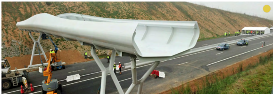
Figure 7.4.22 – Innovative experimental design for a bat passage on the A89 motorway in France. Further research is required to establish effectiveness of such type of devices and define additional landscaping measures to connect the device with bat flight routes (Photo by: D. Riou http://www.denisriou.com/autoroute-a89-chiropteroduc ).
