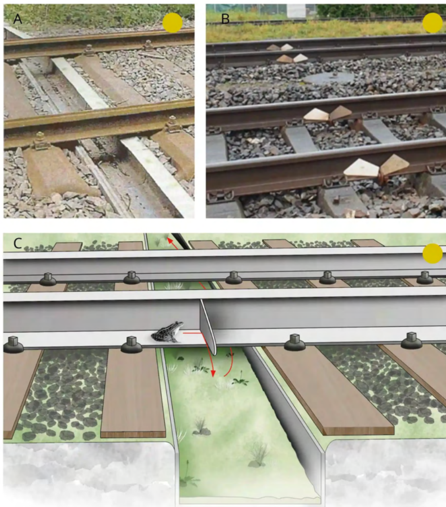
Figure 7.4.55 – Amphibian crossing devices for railways. A: Trench under the railway (Source: Müller and Berthoud, 1994); B: Rejection devices (Photo by: K. Hilfiker); C: Example of the combination of a transversal amphibian barrier in the rail which leads the animal to a trench below. Further research is required to determine the effectiveness of such devices (Source: Iuell et al., 2003 – adapted by AT in 2014 ). ● Favourable; ● Optimal.
