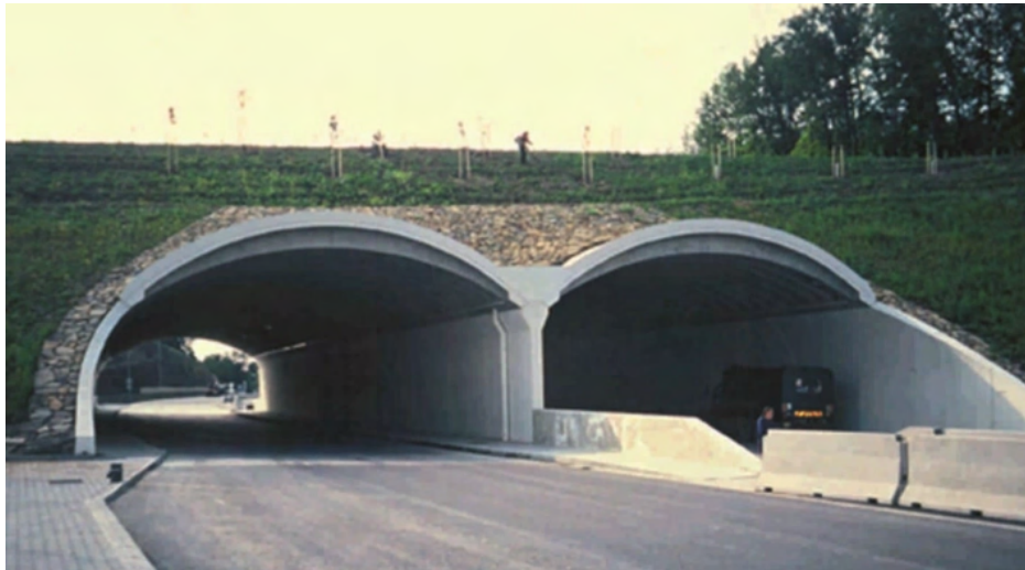
Figure 7.4.12 – Wildlife overpass in the Czech Republic with two prefabricated arches made of concrete (Photo by: H. Bekker).
