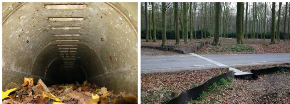
Figure 7.4.54 – Examples of amphibian passages: A: dome-shaped underpass (Photo by: M. Puky) and B: top-grated underpass (Photo by: E. van der Grift). Open grid tunnels are not recommended in all situations as they can suffer pollution from water that drains into the tunnel or from salt in roads located in mountain cold-weather areas.
