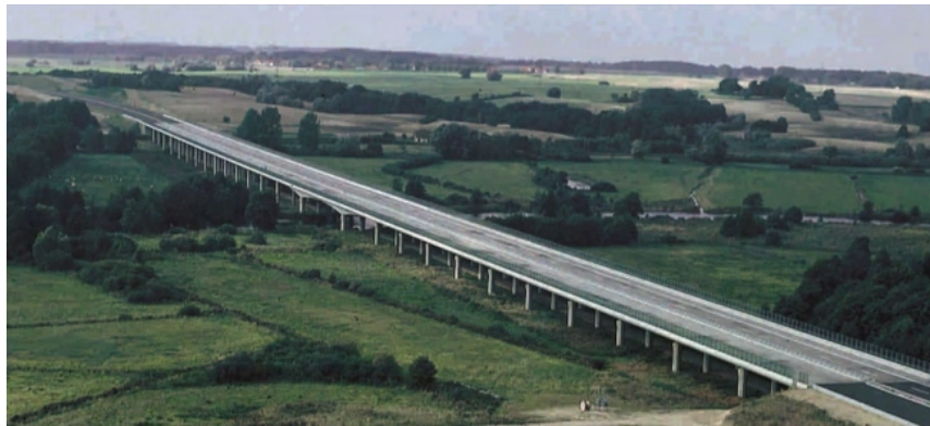
Figure 7.4.24 – Instead of building an embankment, the A20 motorway in northern Germany was built on pillars. This viaduct preserves the floodplain and marshes below and is high enough to allow continuity of vegetation (Photo by: DEGES).
