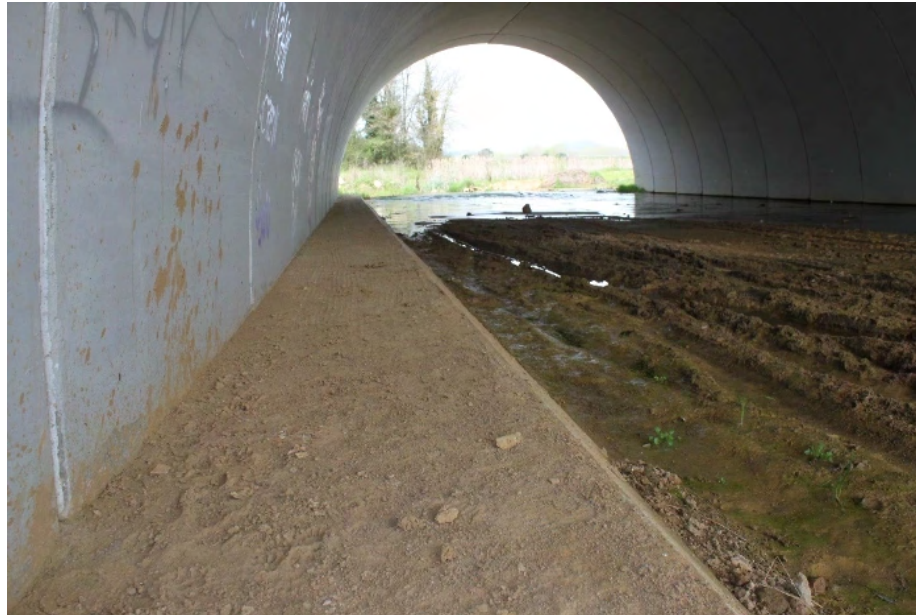
Figure 7.4.41 – Culverts in Mediterranean areas may remain dry or with low water level for much of the year, but require large dimensions for drainage during periods of heavy rain. These structures are particularly suitable for adaptation to wildlife by providing dry ledges, appropriate landscaping at the entrances and guiding fencing (Photo by: Minuartia).
