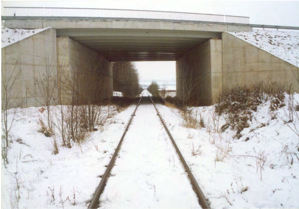
Figure 7.4.36 – Multiuse underpass combining wildlife use and crossing of a low traffic intensity railway. Wide strips of natural soil and vegetation are provided to enhance its use by fauna (Photo by: V. Hlavac).
