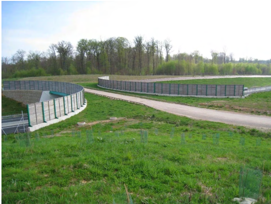
Figure 7.4.20 – Vegetated strips along both sides of a multiuse overpass including a forestry track with very low traffic intensity increase the permeability of infrastructure for wildlife as in this overpass in France. Screens to reduce noise and visual disturbance from traffic circulating under the structure are also installed (Photo by: Cerema).
