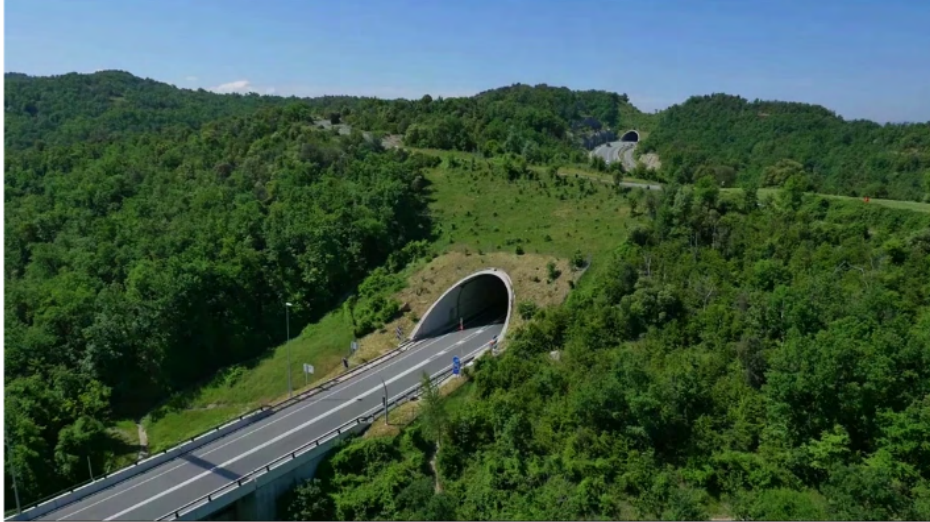
Figure 7.4.14 – Landscape bridges (also known as ‘ecoducts’ and ‘green bridges’) provide optimal opportunities to restore ecological connectivity such as these structures on the C37 in Catalonia, Spain. They also provide a place to deposit material excavated from adjacent areas, reducing the needs to transport for disposal. (Photo by: Minuartia).
