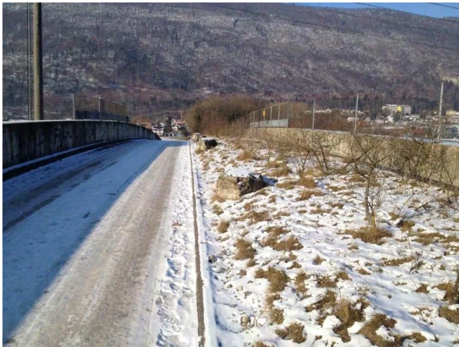
Figure 7.4.19 – A strip of natural soil and vegetation covering a part of the overpass facilitates wildlife crossing, also for small animals. (Photo by: A. Righetti).
