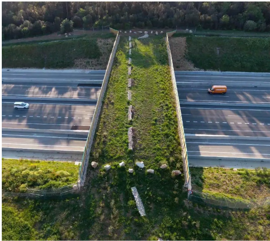
Figure 7.4.17 – Wildlife overpass including stone rows to provide refuges for small fauna and guide animal movement over the passage, vegetation to benefit pollinators and boulders to block vehicle access on the A2 road in Catalonia, Spain (Photo by: Minuartia).
