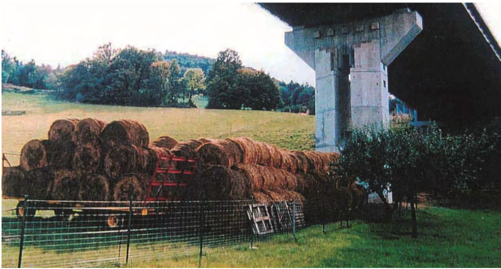
Figure 7.4.29 – Unsuitable uses under the viaduct can prevent animal movement such as this example on the RN59 in France, where a fence and stored material block wildlife access (Photo by: J. Carsignol).
